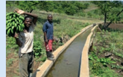
Mulanje Micro Hydro Scheme for electricity generation for households, schools and clinics
