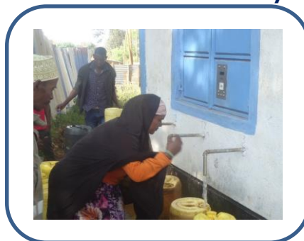
Mrs. Hirbo fetches from a water kiosk fitted with pre-paid water meter- Photo credits Kenya RAPID
