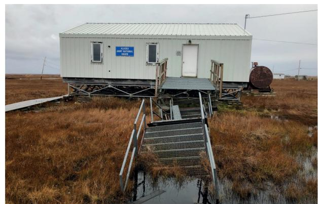
Buildings in Nunapitchuk, Alaska, are sinking due to thawing permafrost, a frozen layer of soil that has underpinned the Arctic tundra and boreal forests for millennia. This thawing ground produces massive sinkholes, forms and drains new lakes, and collapses shorelines already at today's temperatures.
