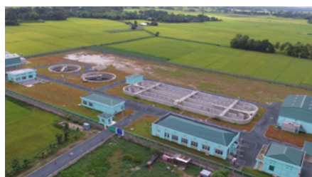
Long Xuyen sewerage, drainage and wastewater treatment system project in Vietnam
