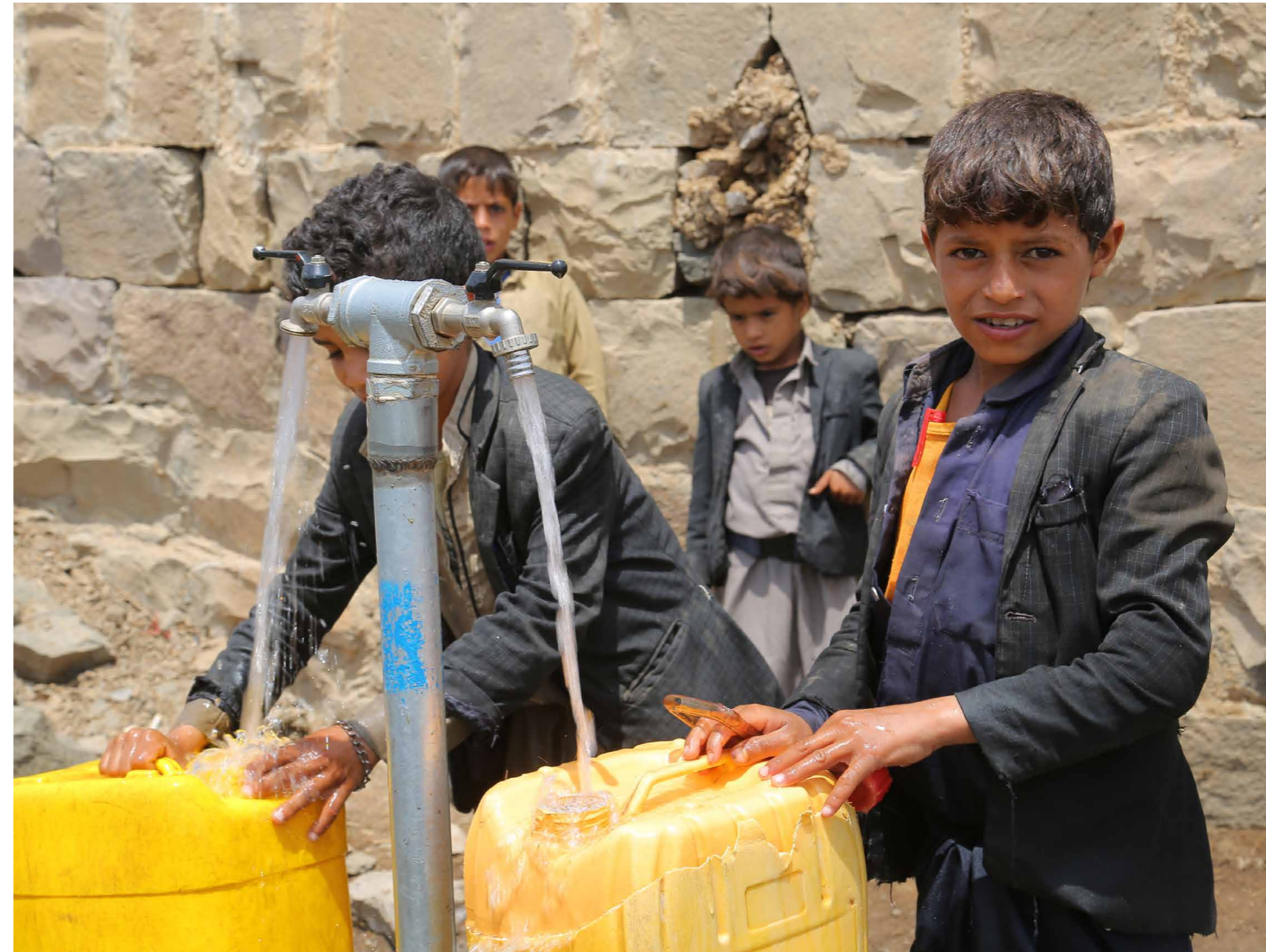
In Sana'a governorate, boys collect water from a facility repaired by Islamic Relief as part of our response to the dire and deepening crisis in Yemen.
