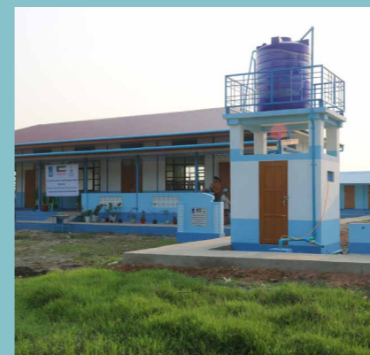
A school in Kan Chaung village, Myanmar, renovated by Islamic Relief. We added three classrooms, toilets and new school furniture. Safe drinking water and a new entrance road were also provided, supporting children to continue their learning in a safe and suitable setting.
