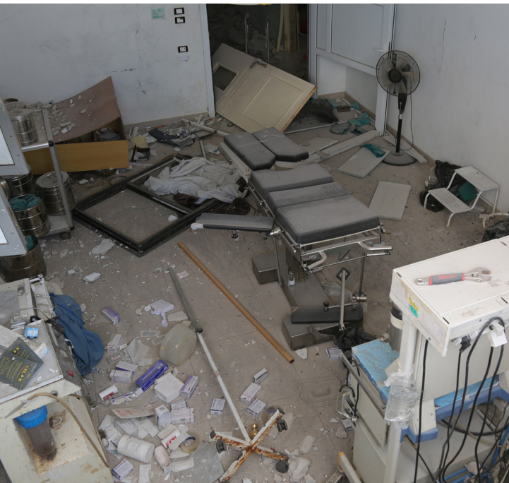
In 2018 Al Rahma Hospital in northwest Syria was completely destroyed by an airstrike, leaving it out of service. PHOTO: frontlineinfocus
