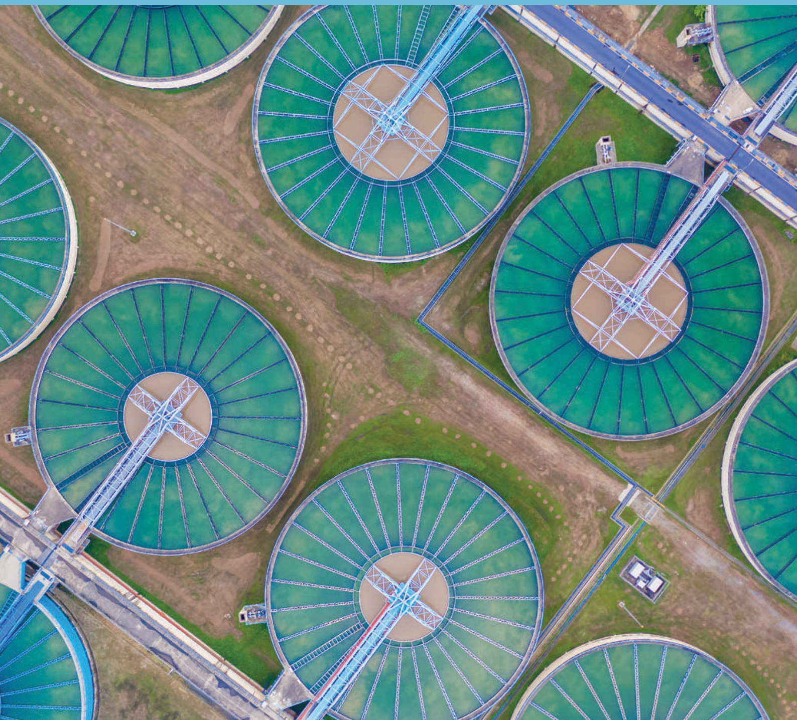
Aerial view of a water treatment plant.
