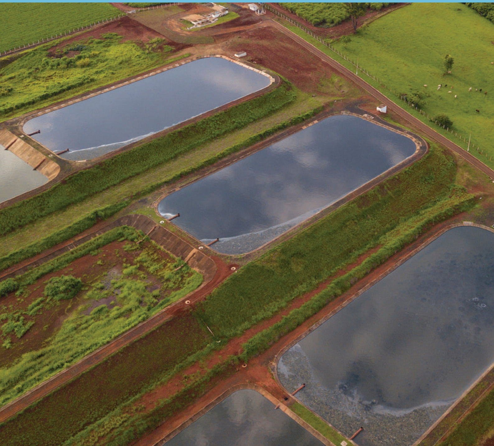
Aerial view of a sewage treatment facility.
